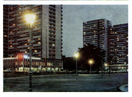
The lighting project of the street 'Leninallee' in the county town Halle/Saale is performed as high column installation of 24 m in height. Each column is provided with 12 side-entry fixtures equipped with the high pressure sodium lamp type NA 400-01. Figs. 16 and 17 demonstrate this lighting installation seen from the same view point, firstly in direction to the highway and than in the opposite direction.
