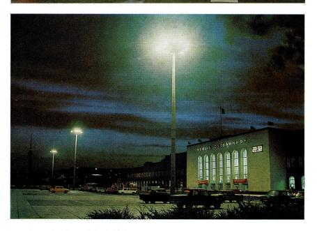
The lighting of the parking lots at the 'Berliner Ostbahnhof' is provided by three 24 m columns equipped with rectangular mounting supports. Twelve fixtures with one NA 400-01 lamp are arranged on the top of the column (Fig. 12). The station building itself is also illuminated by this lighting system and exhibited by its high illuminance.
